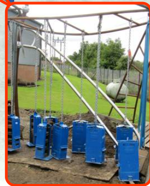
Monkey Bars structure and weight test
